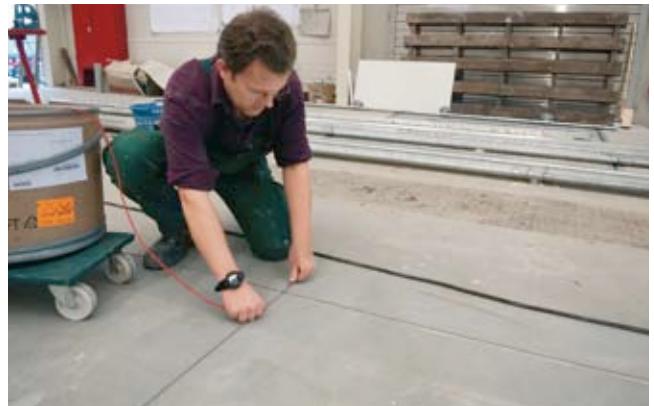
Inserting the cable
